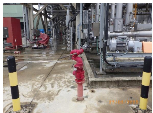
Fire Water Hydrants with Water Monitor
