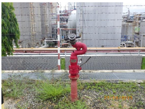
Fire Water Monitor with Foam Induction
