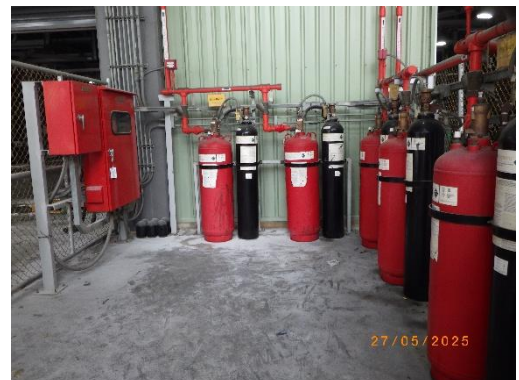
CO 2 Extinguishing Systems
